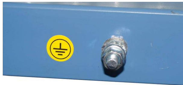
Fig.: The spot for the machine's grounding
