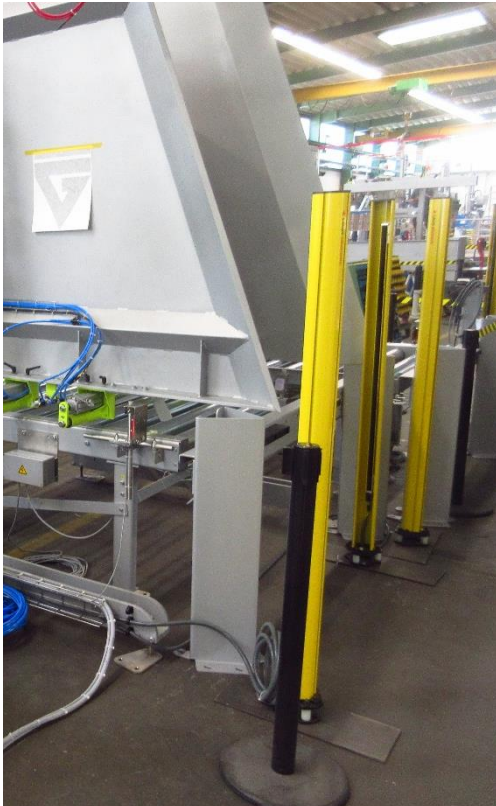
Figure 7 Safety light curtains (7)
