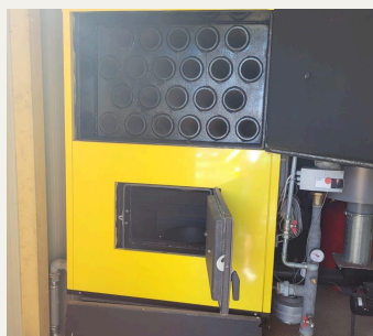
Fire-tube HX with turbulators
