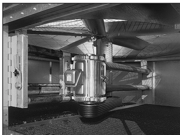
Motor Base Assembly
