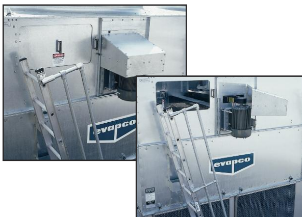
External Motor Mount (with optional ladder)
