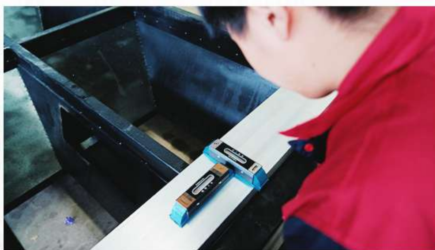
Bed Foot Installation
