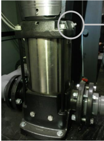
Figure 17: Position of the pump vent (vertical type)
