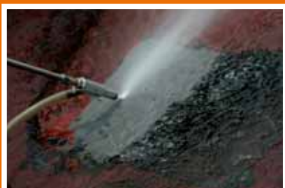
Surface - Sand blasting
