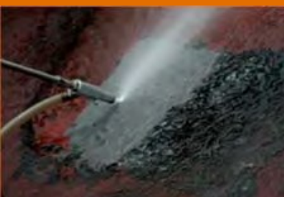
Surface sand blasting
