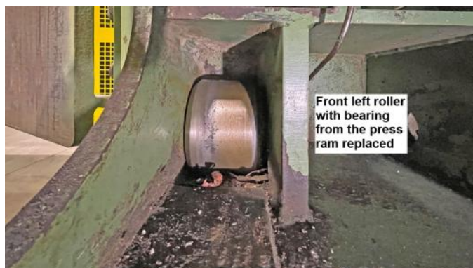
Main hydraulic cylinder dismantled, disassembled, checked, cylinder barrel honed, seal sets replaced, final assembly, pressure test carried out.
