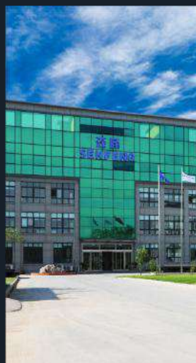
Production base (Lingang Road, Jinan City)
