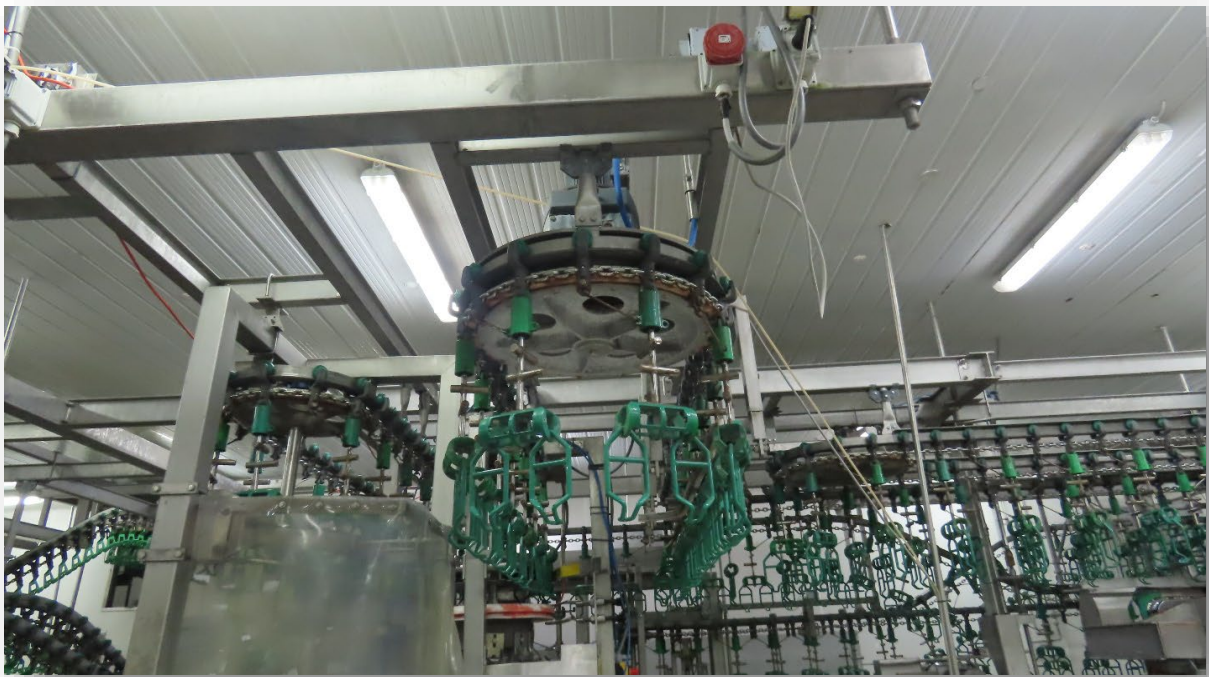
Picture 23: Support structure: OHC, drives, hangers
