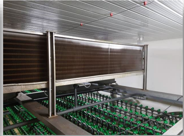
Picture 6: Tunnel with liquid ice unit
