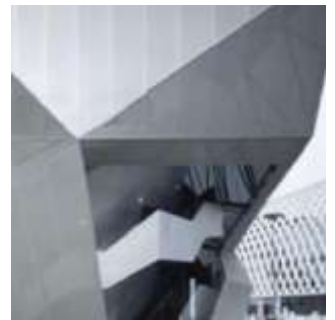
Decorative curtain wall
