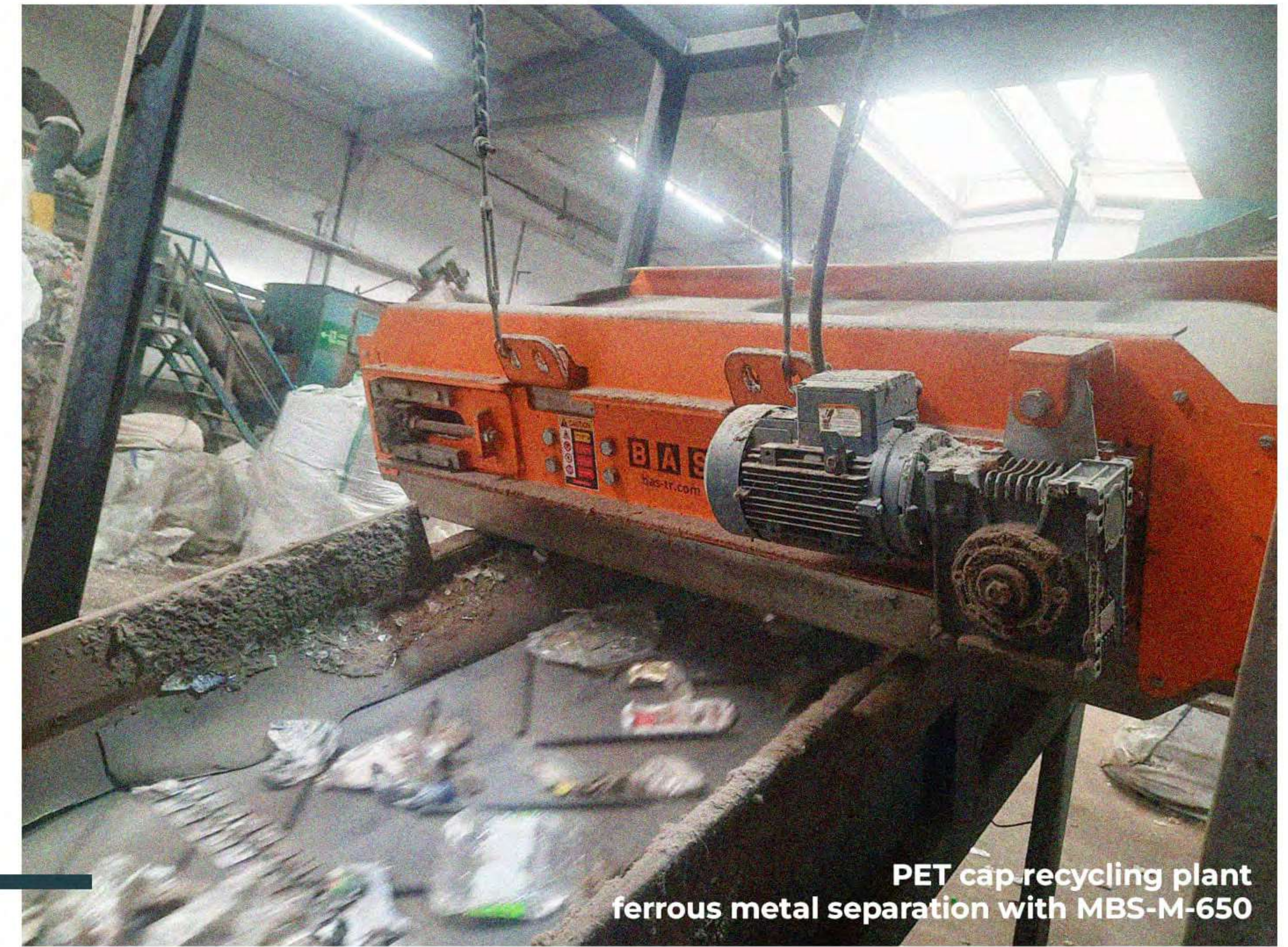
Casting plant ferrous metal separation with MBS-M-1000 over the sand conveyor
