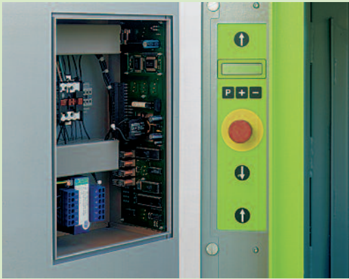
Low-maintenance: Microprocessor control
