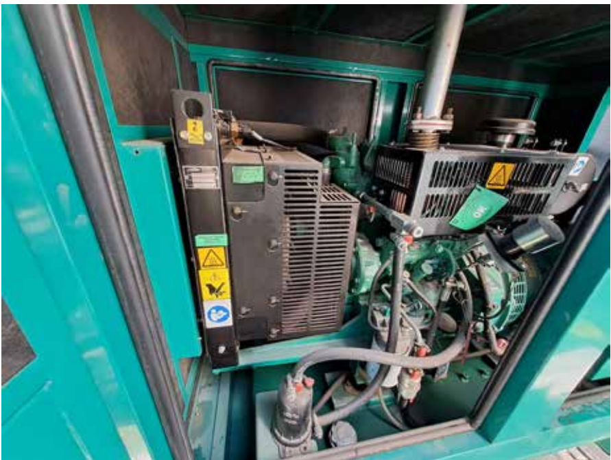
Lot. 31: CUMMINS 25/20 KVA /KW Generator, Model C20D6, Serial Number D21I1150171, Year 2021, Voltage 220 V, 60 Hz, 1,317 hours of use, Made in India.
