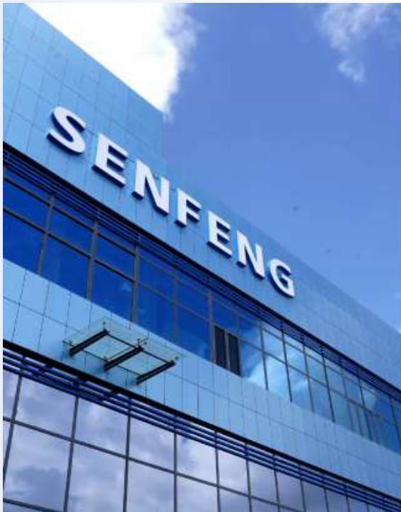
New Headquarters Base (Jinan High-tech Zone)
