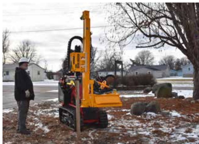
Installing 3" Round Wood Fence Post.
