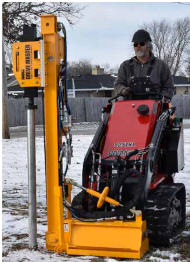
Installing 2 3/8" Terminal Fence Post.
