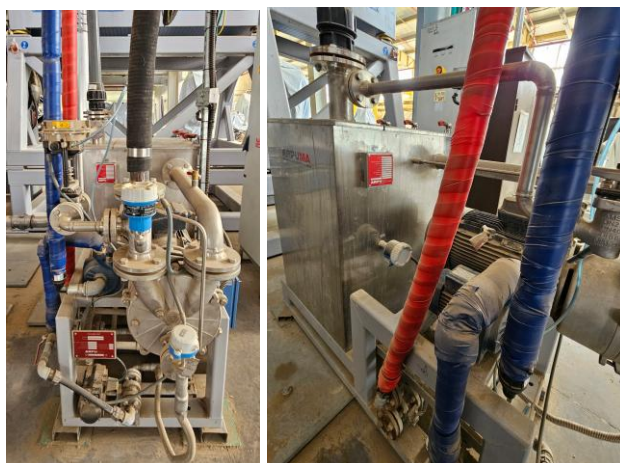
Left: vacuum pump Right: vaccum pump tank
