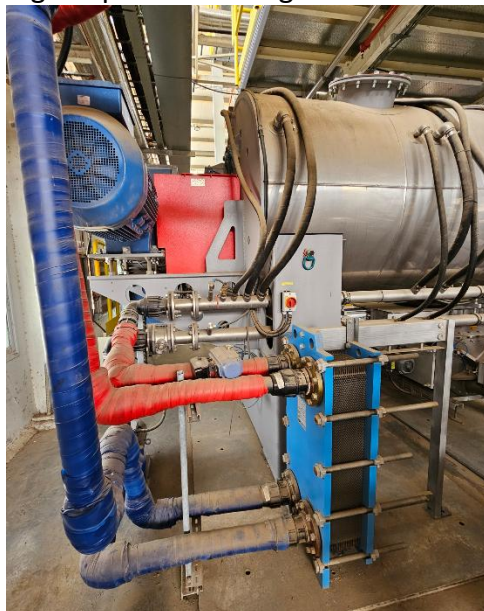
Left: drive of the mixer and cold water – cooling water - installation Right: Type plate cooling mixer
