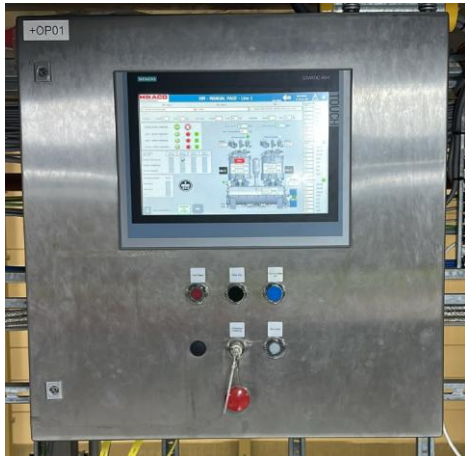
Left: HMI hot mixer Right: main page hot mixer (from main plant with two Hot mixer)
