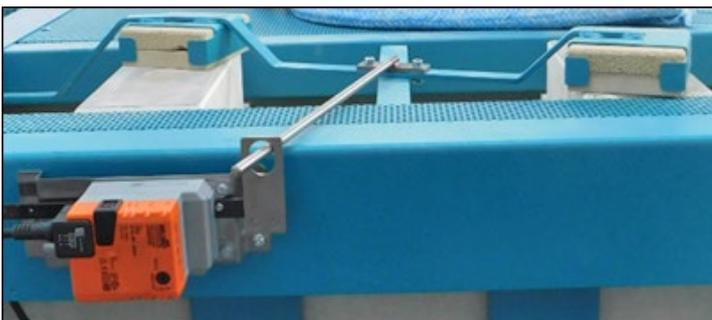
Figure 25: Automatic exhaust air flap
