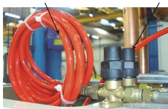
High pressure Lines ready to be connected to the valve
