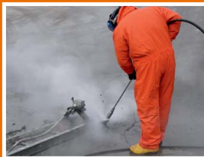
Removing concrete.
