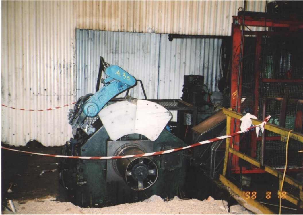
1. Tandem Mill Uncoiler
