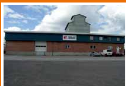
DEN-JET Factory Denmark.
