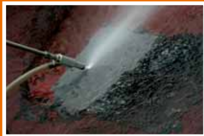
Wet Sand-blasting on Corroded steel plates.
